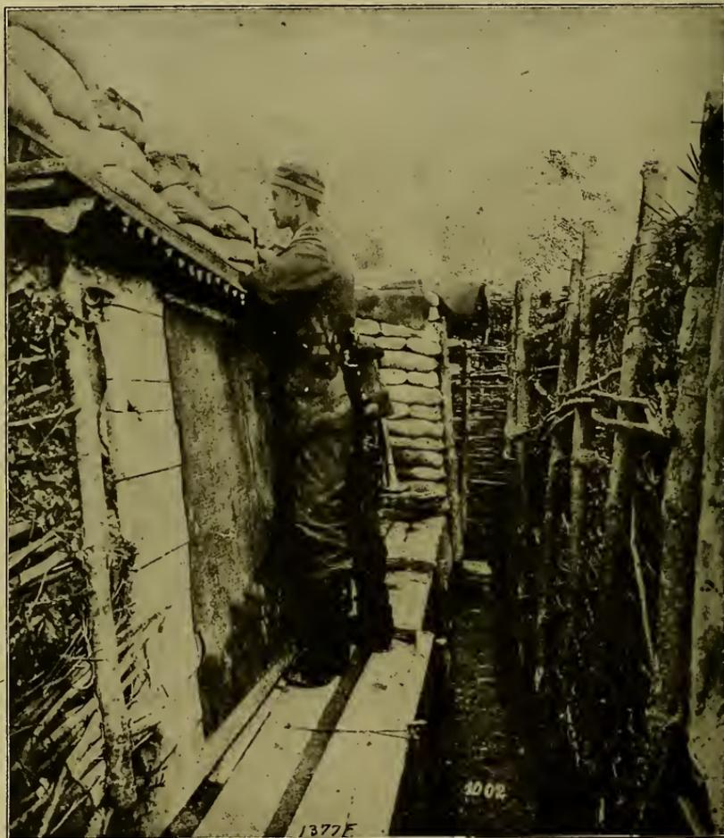
A German Lookout in a Waterproof Trench. A view of a sandbag-constructed trench on the German battlefield in the Western battle zone showing how carefully the trench has been water-proofed.
